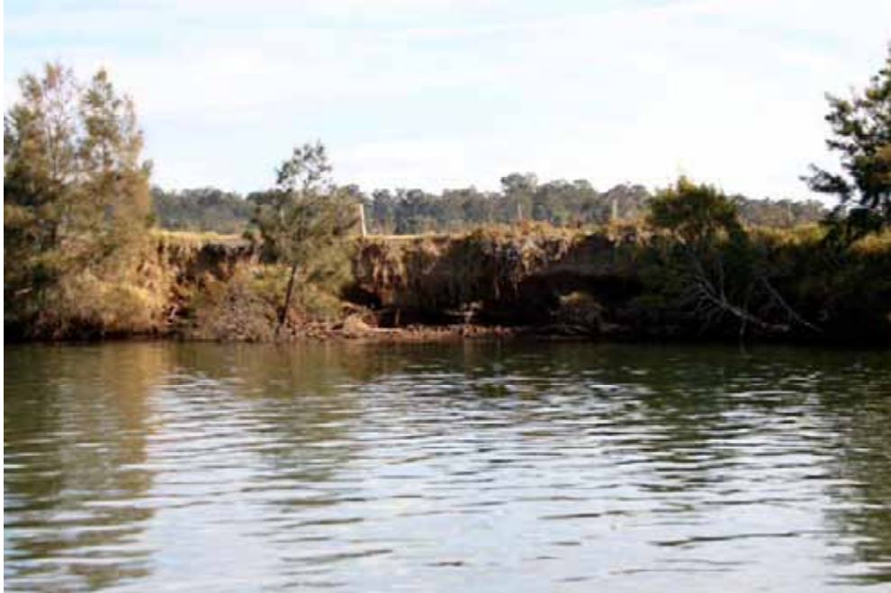
Outside bend erosion
